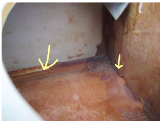
Figure 2. Damaged Fillets.
